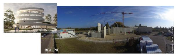
After completing the foundations, the first sections of the curved concrete walls leading from the hall of the future spiral to the scenographic space were built. This was followed by the triple-level walls which are almost 8 meters high. Its white-tinted facades were poured in one go and will form the periphery of the base. A few weeks ago, the prefabrication of the hemp concrete insulating modules began. The next step will be the installation of the roof structure.
